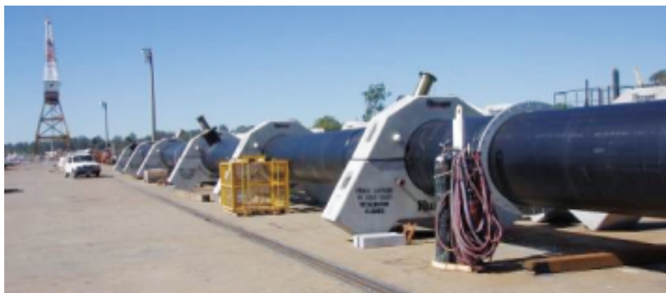
Figure 8. Concentrate Discharge Diffusion Structure (Photo courtesy of Sinclair Knight Merz)
